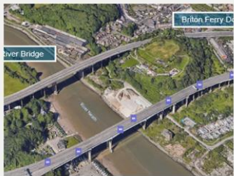
Case Study: Reliability-based Assessments for South Wales Trunk Road Agent
