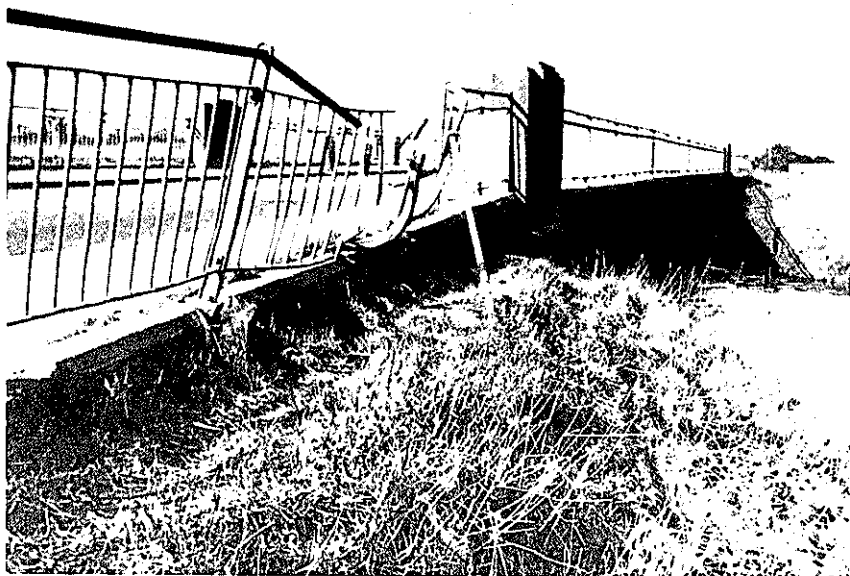
Plate 23. Damaged parapet due to impact
