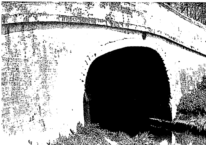
Plate 16. Distortion of arch profile
